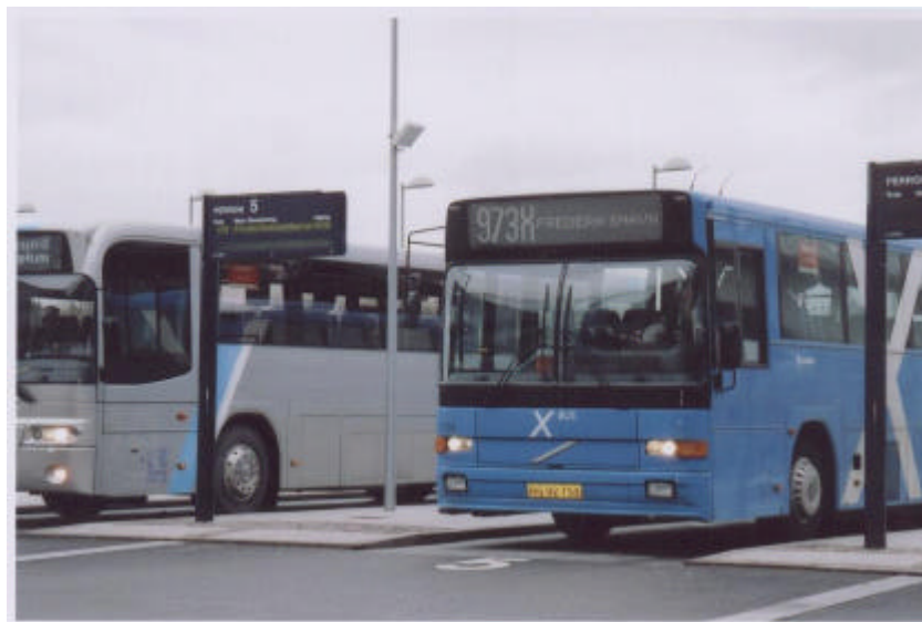
Fig. 6-6 Aalborg Compact Bus Station
